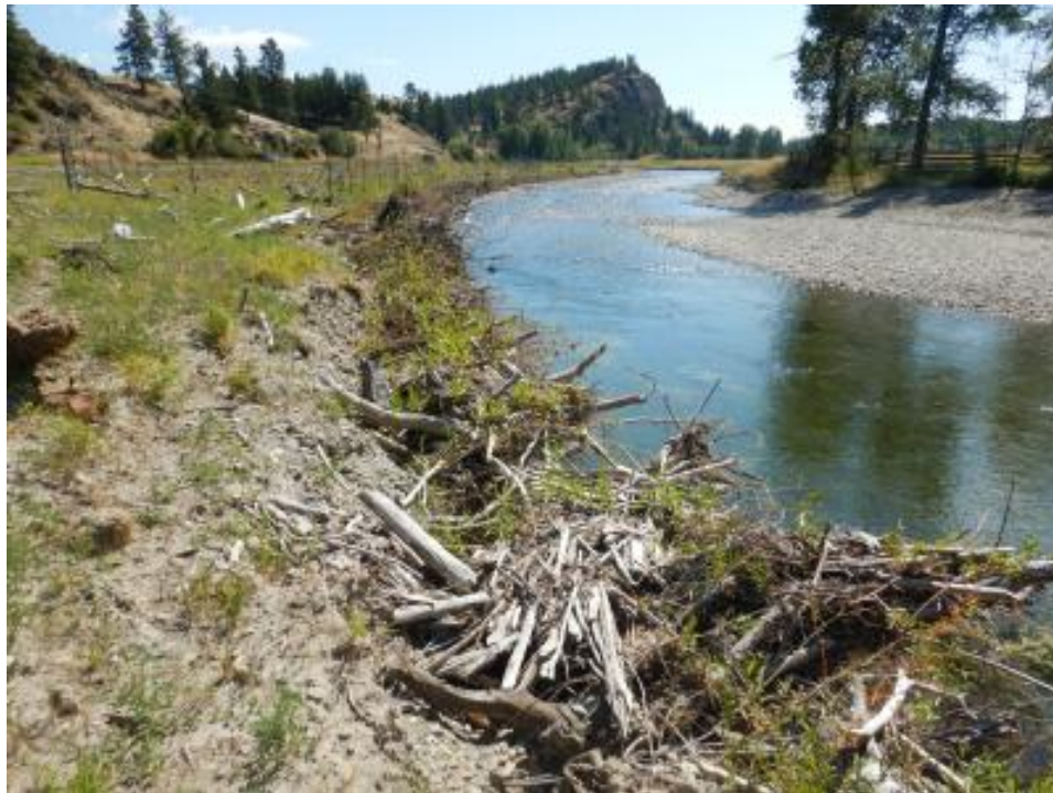
This post-project photo shows bank stabilization using woody debris and willows (photo by Lincoln CD).
