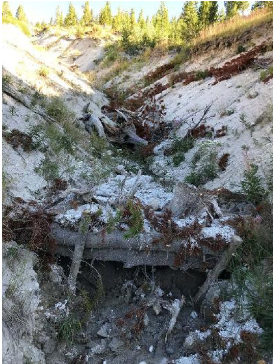
Examples of gully check dam structures that capture sediment pollution (photo by BHWC).
