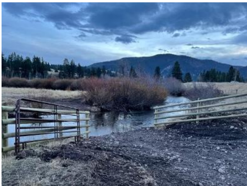
A portion of one of three projects implemented under the Ranching for Rivers program in 2021, before (above) and after (below) a water gap was installed on Cottonwood Creek (photo by Blackfoot Challenge).
